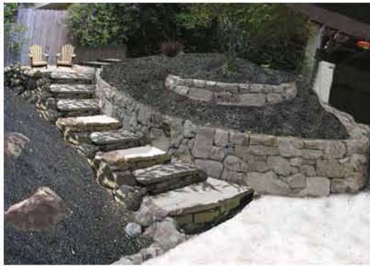
Showing the hardscape alone allows the clients and contractor to clearly see the shapes and textures, as well as plan construction phases. (Photo courtesy of Leigh Designs)
